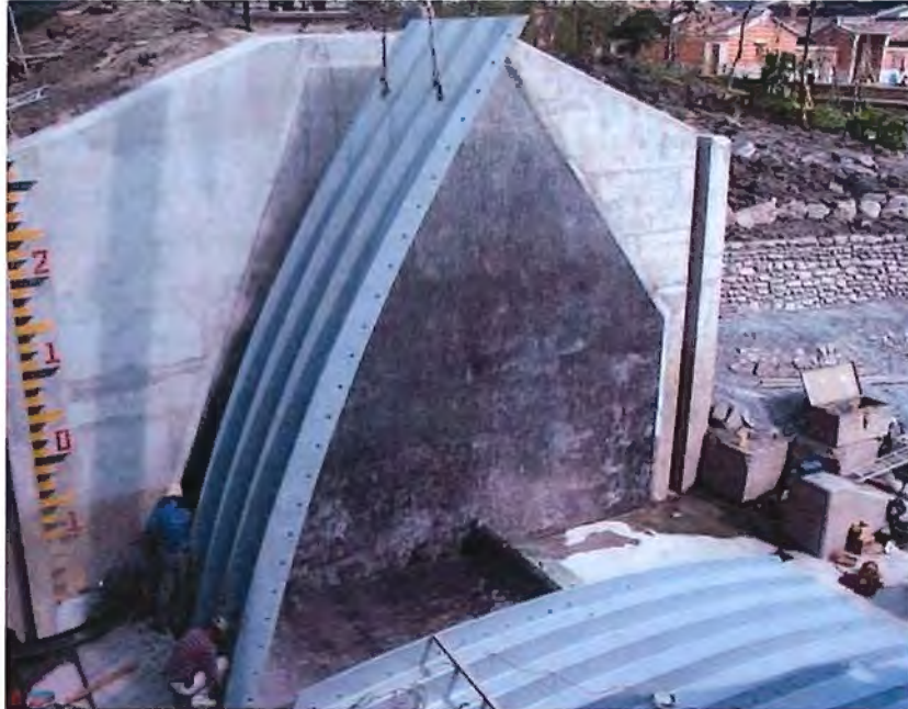
Figure 1-3: Typical Obermeyer Crest Gate Configuration (during installation)
